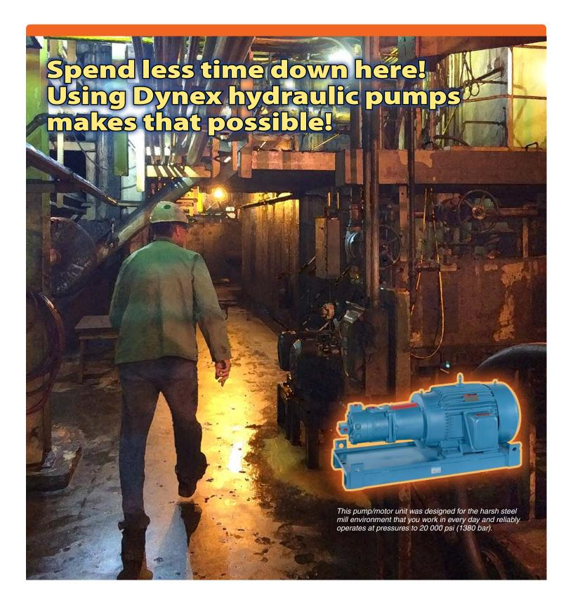
Dynex pump/motor units provide long service life on roll balance and bearing lube systems in harsh steel mill environments. Dynex pumps are ideal because of their exceptional tolerance to contamination and high temperatures. They can provide the performance and reliability of a triplex pump at about half the cost.
